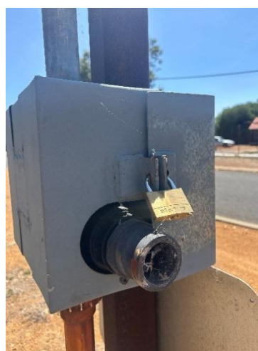
Lock to access standpipe
