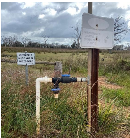
Standpipe detail
