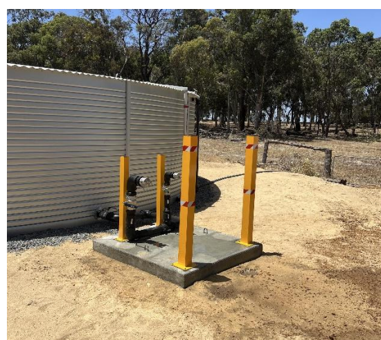
Manifold (50 & 80mm camlock outlets)
