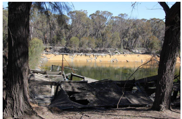
Figure 5: Collapsed Asbestos Roofing
