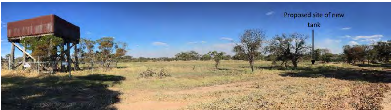
Figure 3-2 Kylie Dam and Proposed New Tank Location
