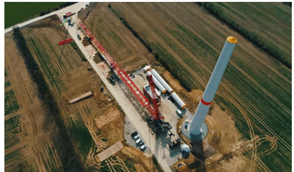
Figure 23: Turbine Erection Process
