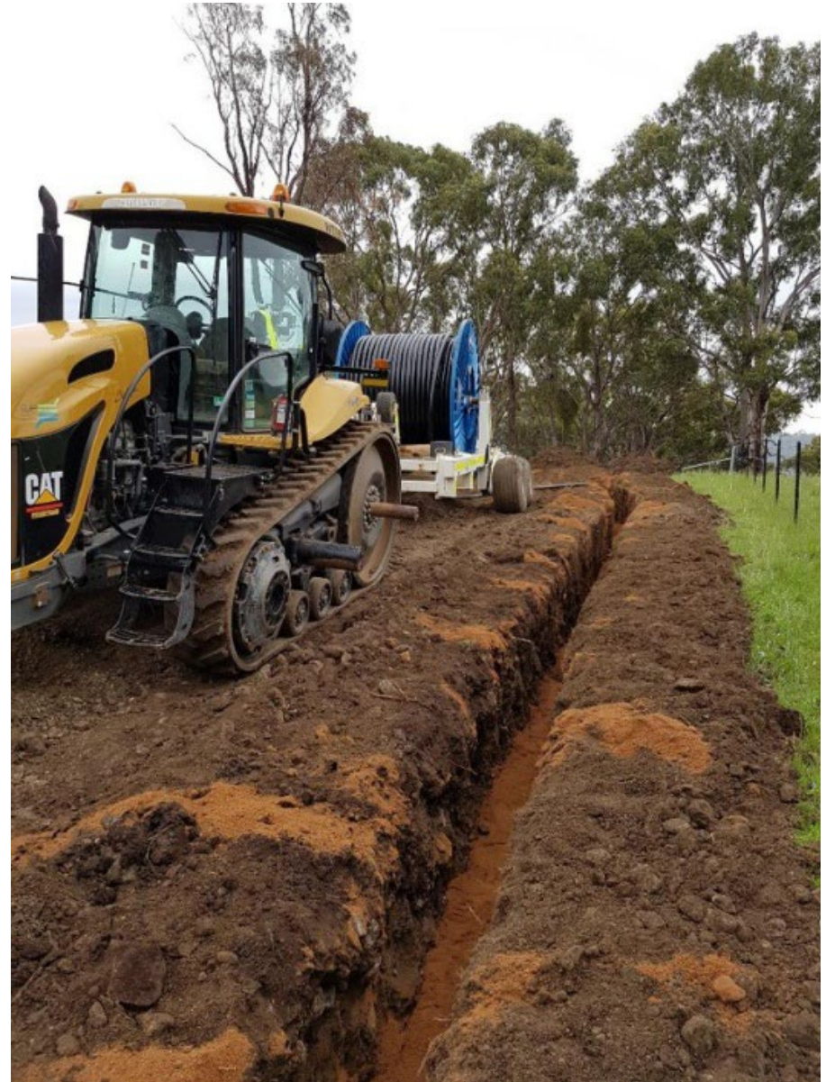
Figure 10: Example of Underground Cabling being Installed
