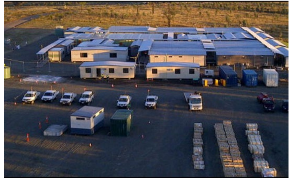
Figure 20: Example of Site Offices
