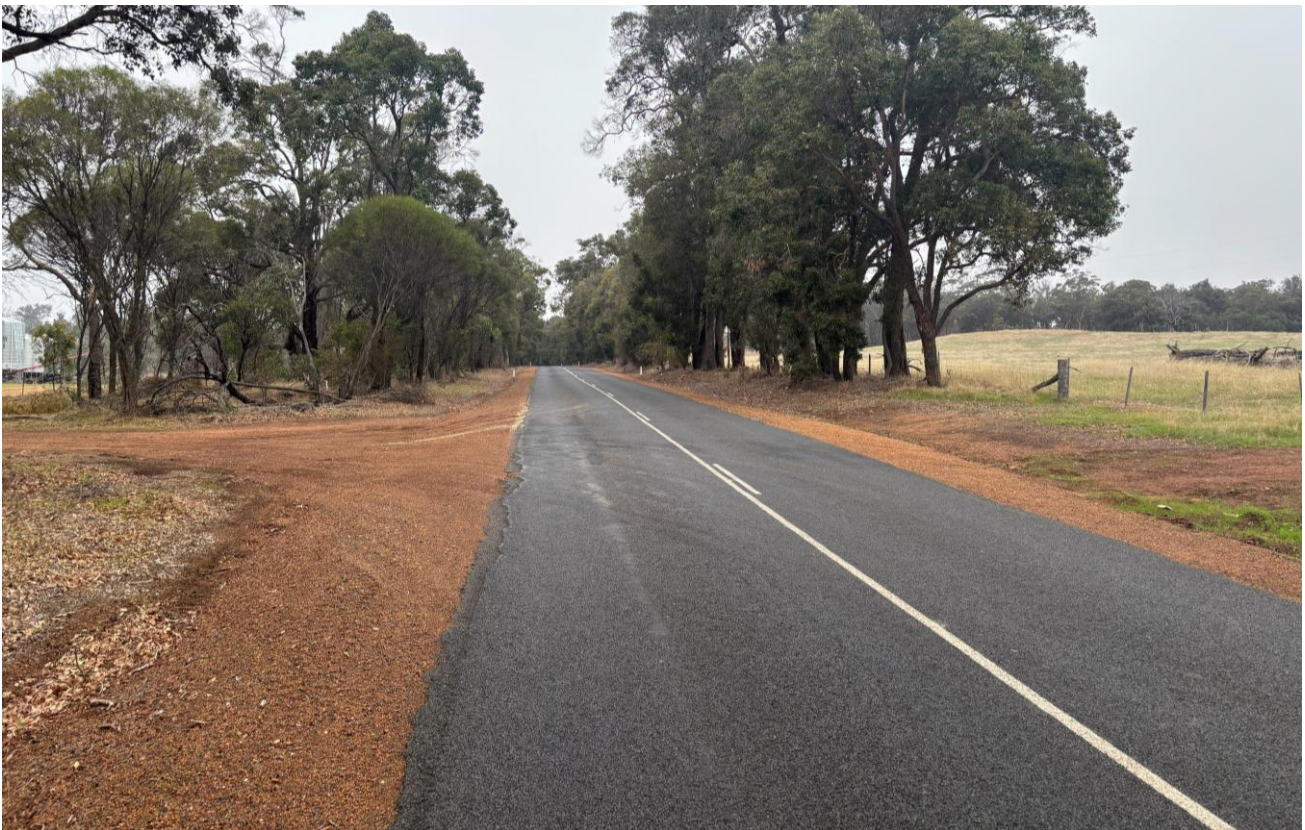
Figure 77 Crossing of Darkan Road – 4.3km from Coalfields Road (source: Flyt)
