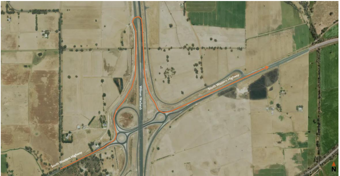
Figure 17 Route along South Western Highway through Wilman Wadandi interchange (source: Metromap)
