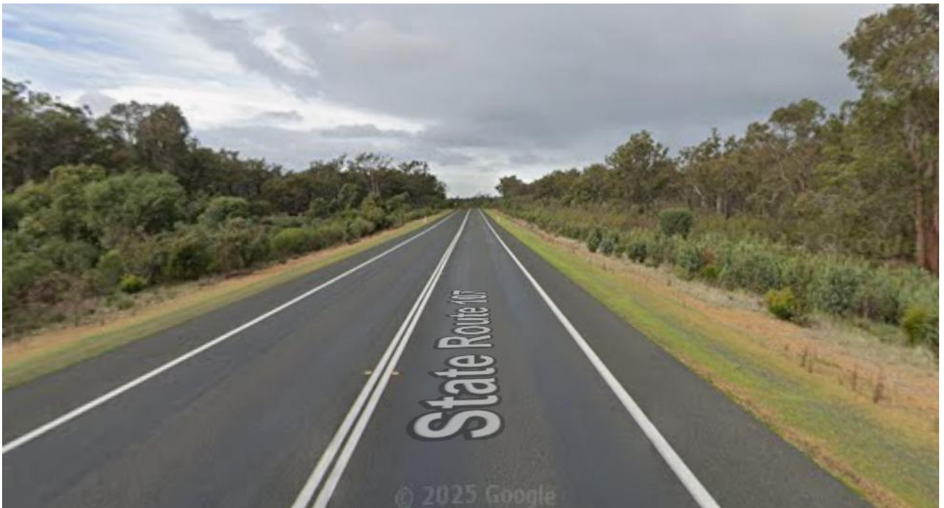
Figure 56 Coalfields Road approximately 700m west of Cordering Road North looking east (source: Google)
