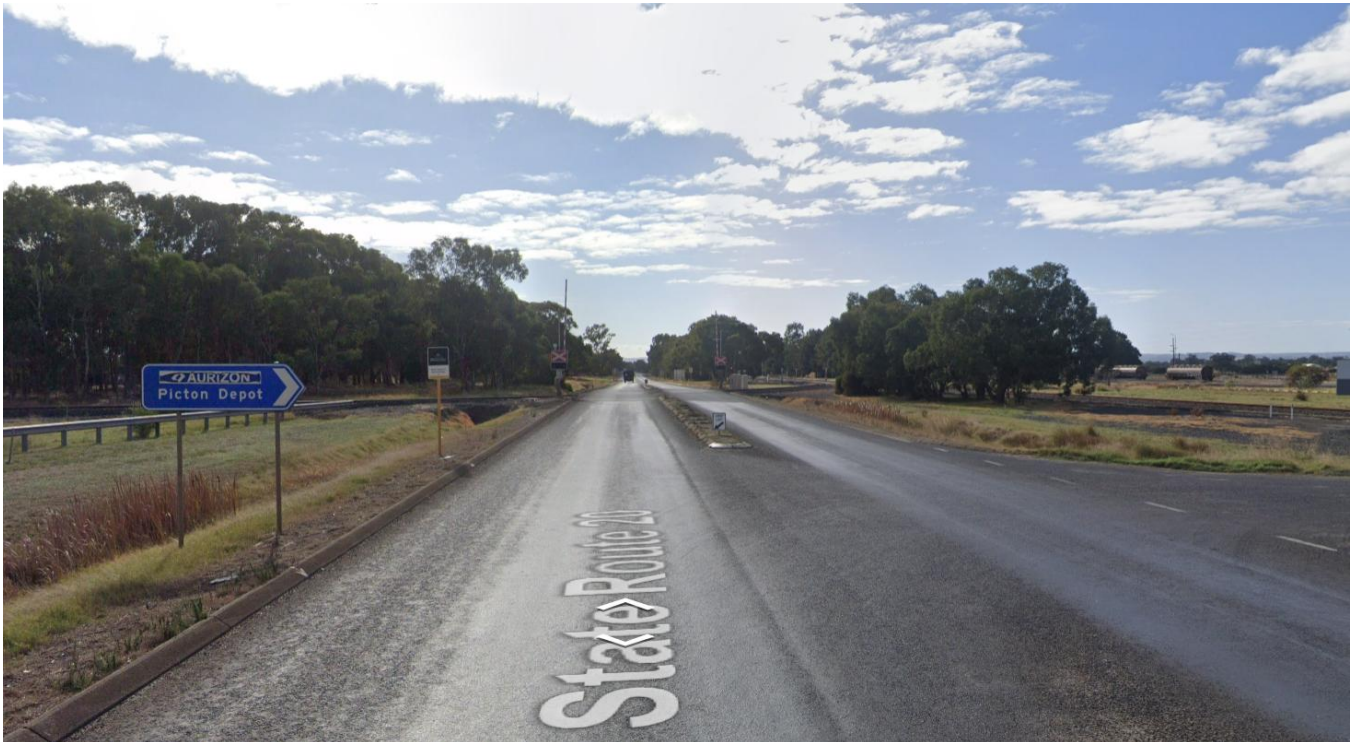
Figure 26 South Western Highway rail crossing (source: Google)
