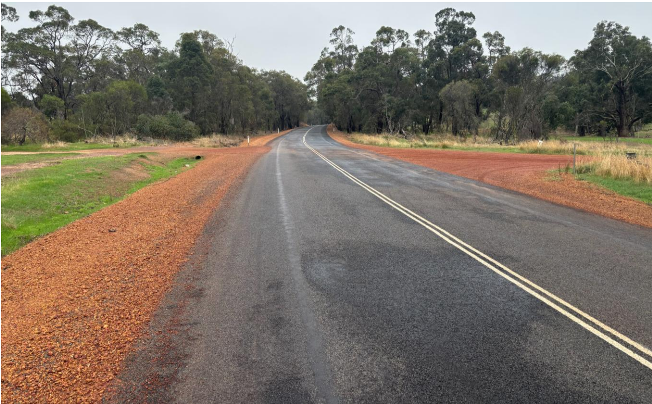
Figure 79 Crossing of Darkan Road – 5.3km from Coalfields Road (source: Flyt)
