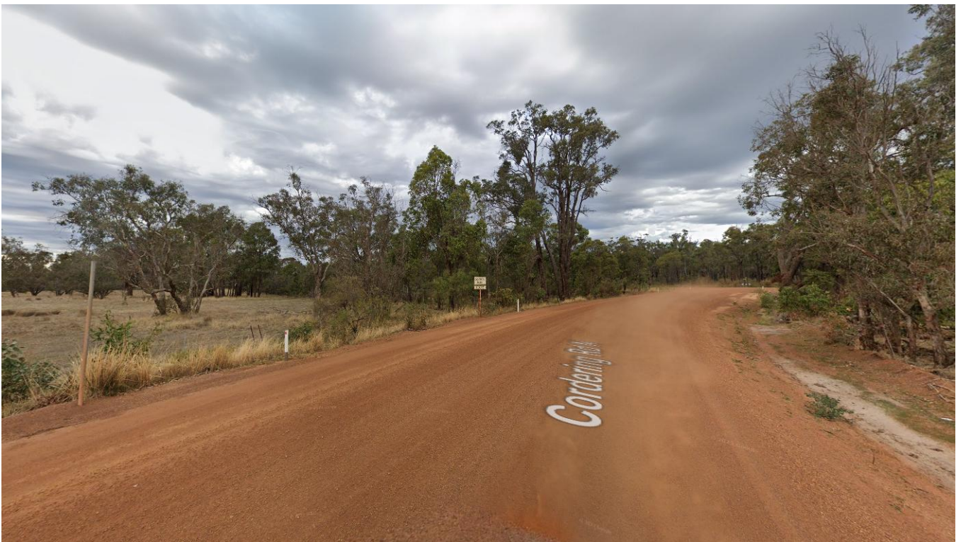
Figure 76 Proposed transmission line access point - CR10 (source: Google)
