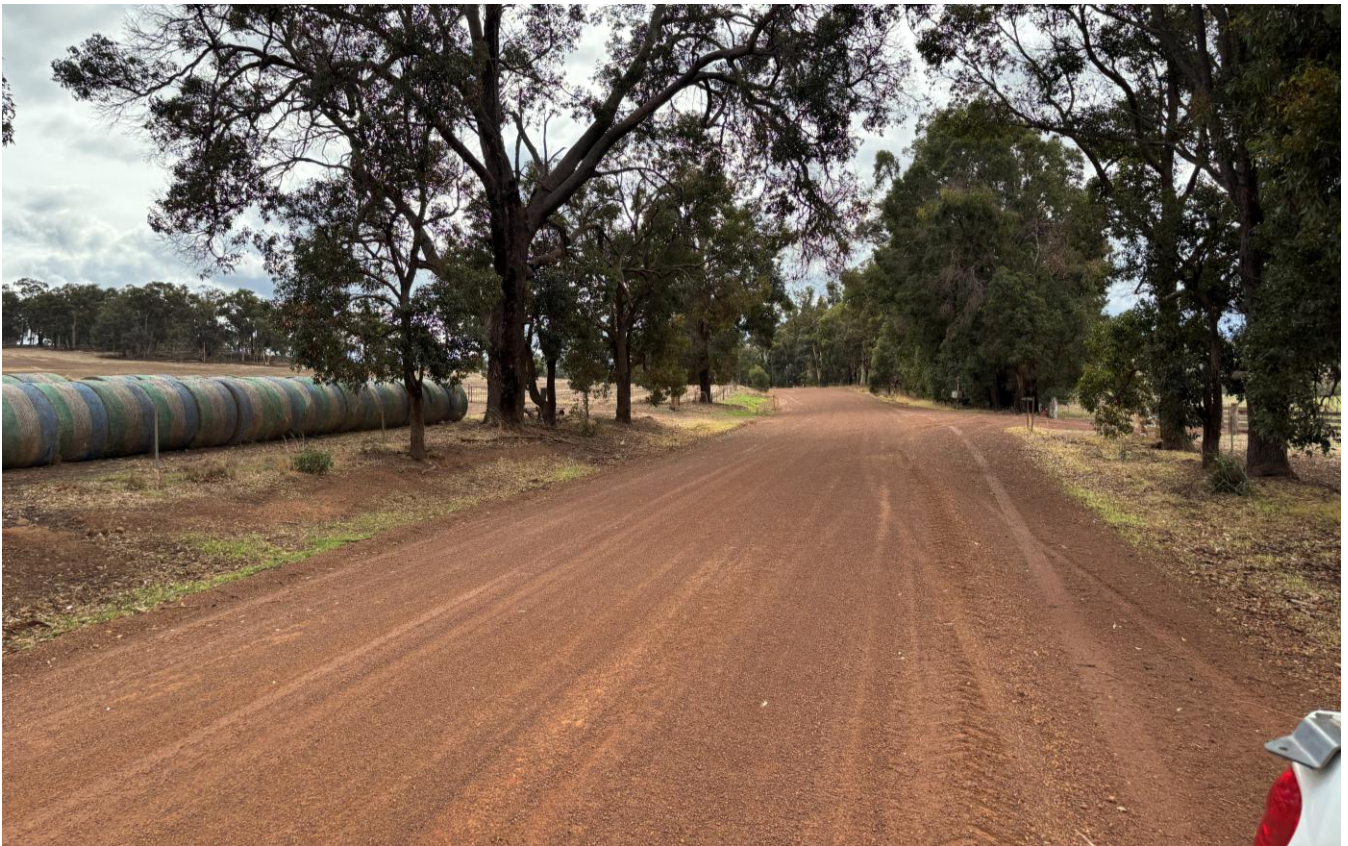
Figure 71 Crossing of Cordering Road North - 9.8km from Coalfields Road (source: Flyt)
