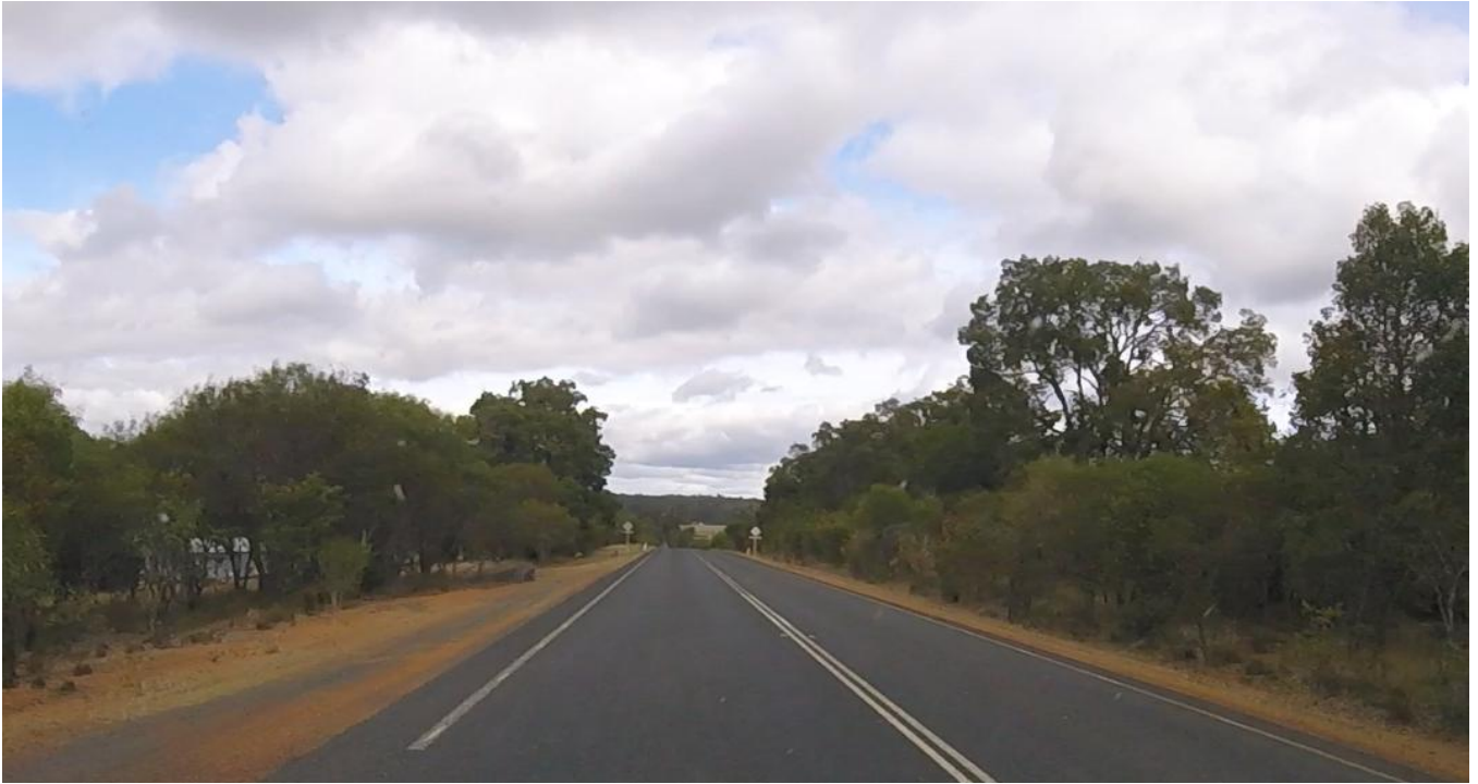
Figure 60 Cordering Road North south of Coalfields Road intersection looking south (source: Flyt)
