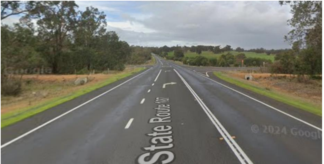
Figure 57 Coalfields Road immediately west of Cordering Road North intersection looking east (source: Google)
