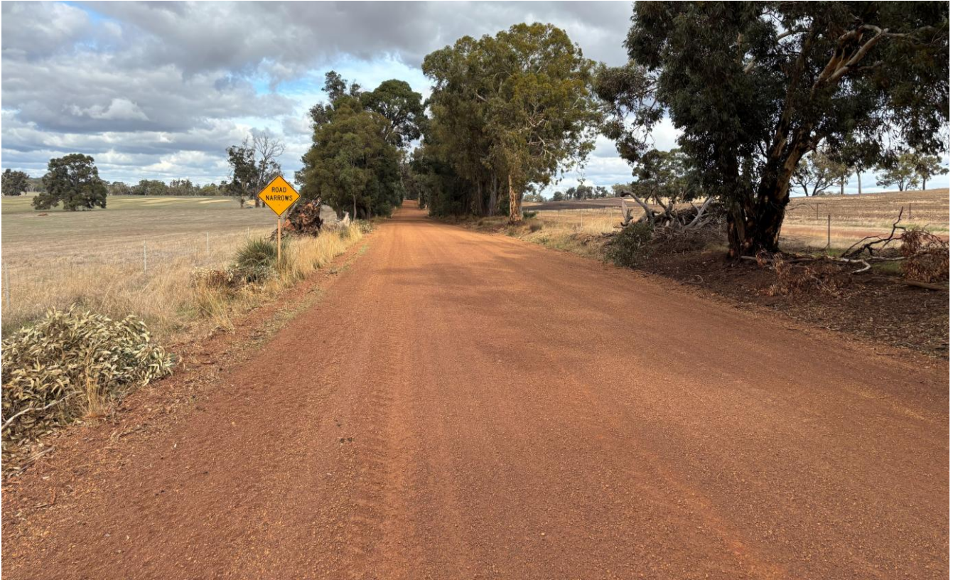
Figure 72 Crossing of Cordering Road North – 10.8km from Coalfields Road (source: Flyt)
