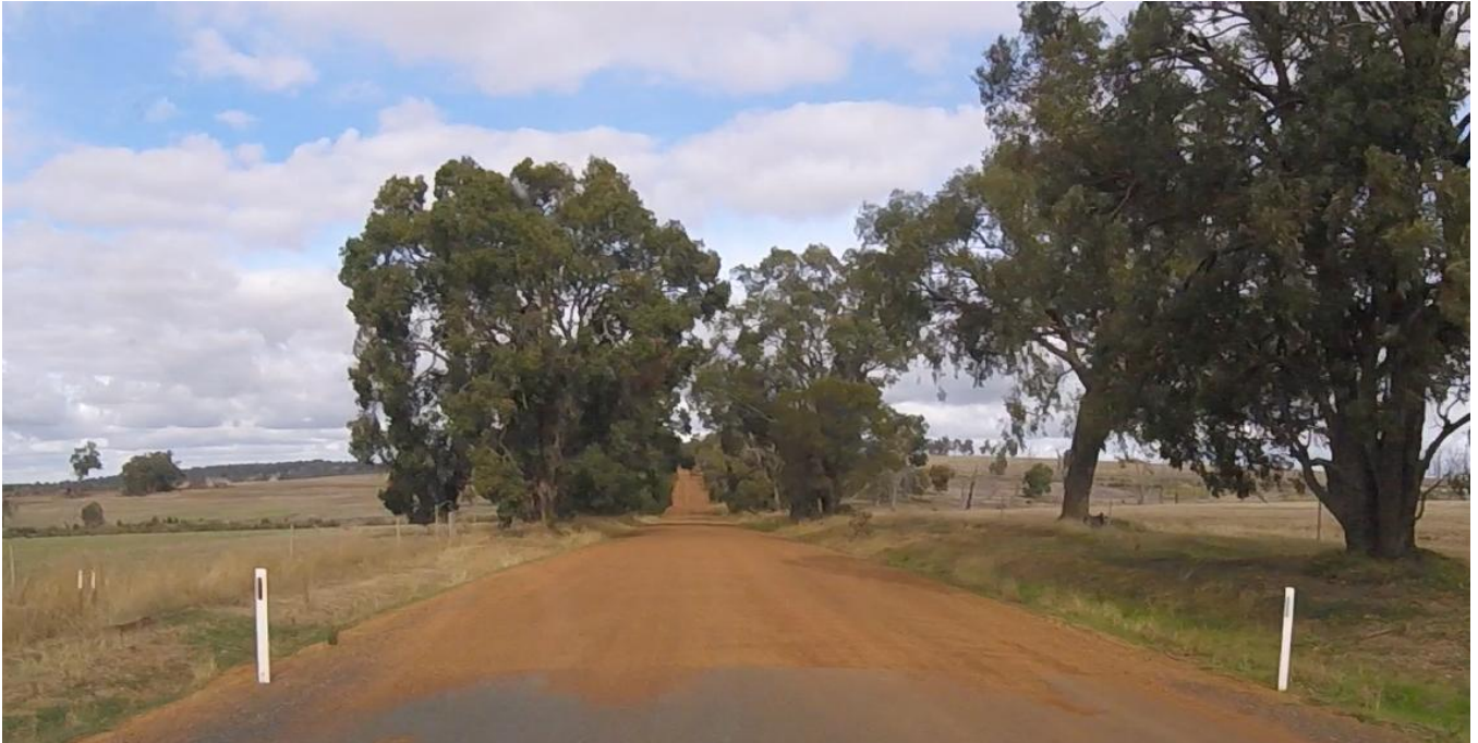
Figure 62 Cordering Road North transition from bitumen to gravel surface (source: Flyt)
